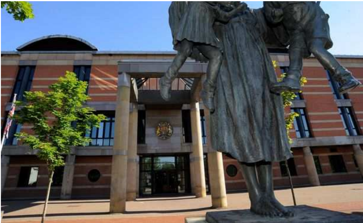
Teesside Crown Court
